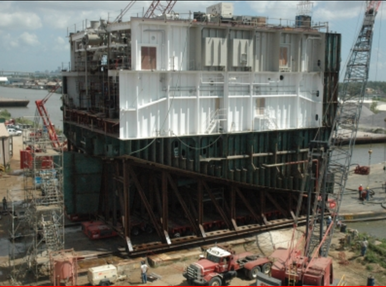
The 1600 ton power module loaded out in Harvey Louisiana.
